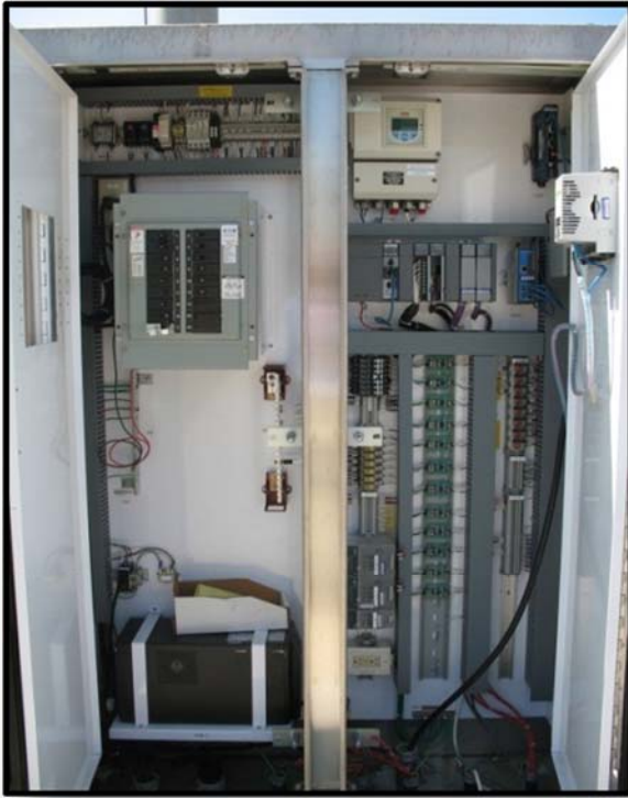
San Sevaine Turnout control panel
