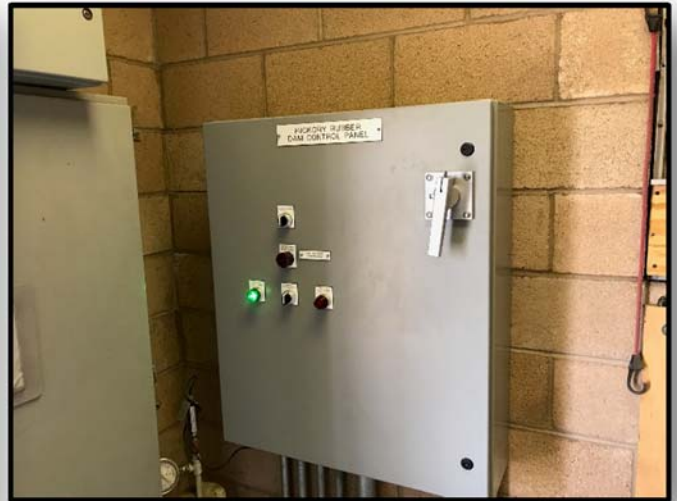
Rubber Dam control panel
