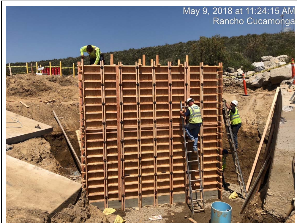
Concrete forms for storm water inlet structure
